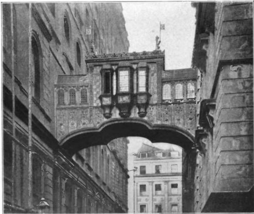
Covered Bridge of Iron, Sheathed in Cast Lead, Grand Hotel, London. Designed by William Woodward, and executed by Starkie Gardner and Co.
